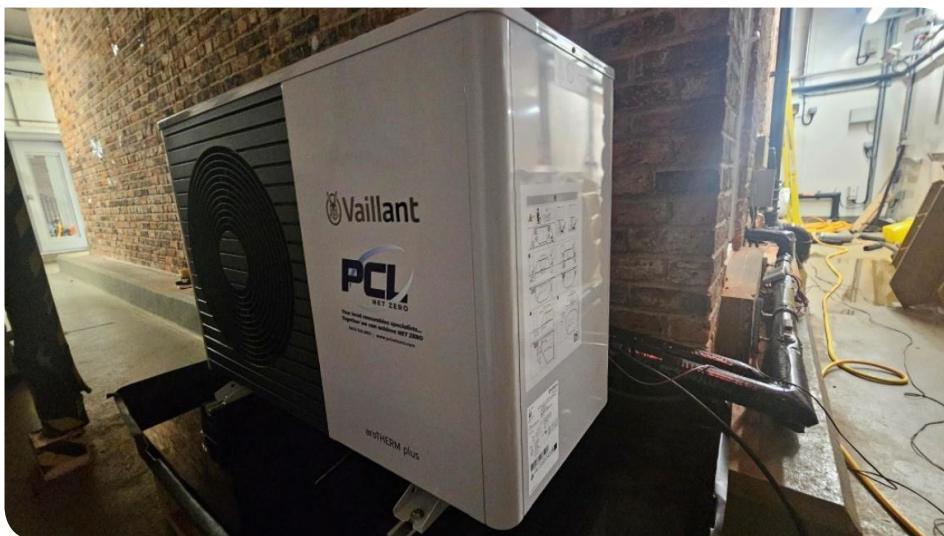
Salford Energy House heat pump installation
